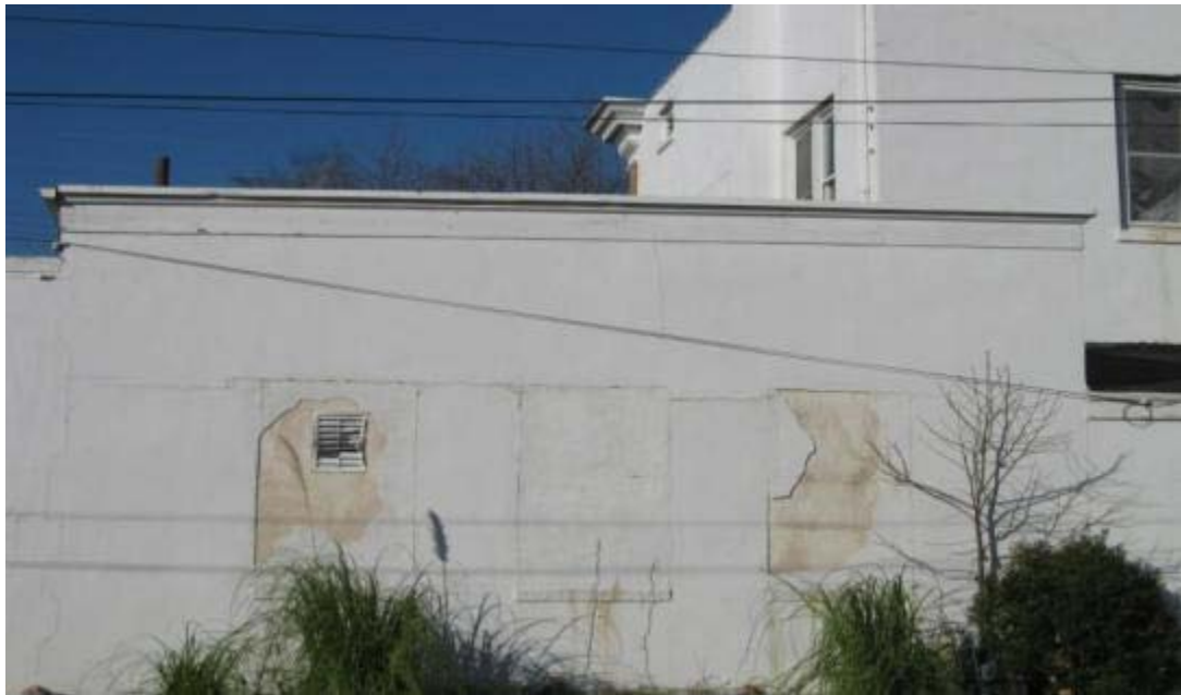
South facing exterior wall
